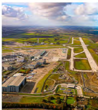
Mark Meehan. North runway Dublin Airport (Ireland).
